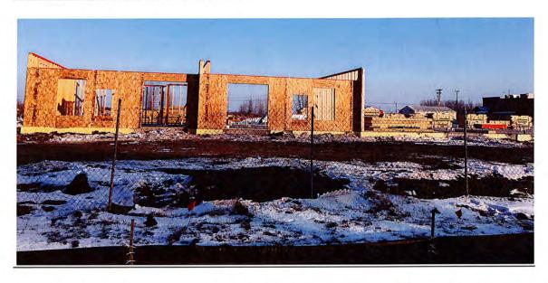
The pace of construction is picking up at  $15^{th}$  Street Flats. The walls for the first floor started going up the end of last week (the photo above was taken 12/9/18). The photo below (12/12/18) shows an enclosed area for the elevator shaft.
