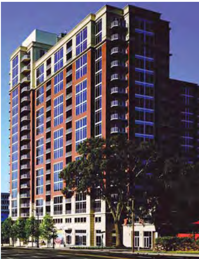
Atlanta's Brookwood condo installed its own fiber backbone.
