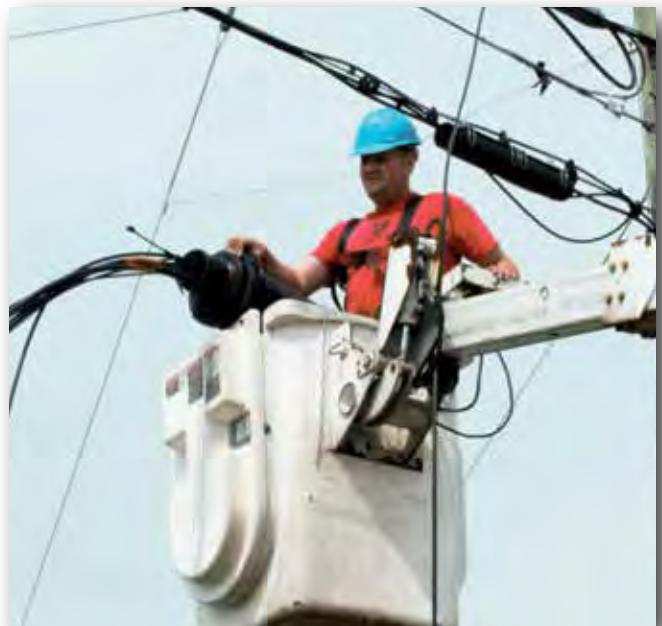
Danville, Va.'s use of its own utility poles for the nDanville network saved the city time and money.
